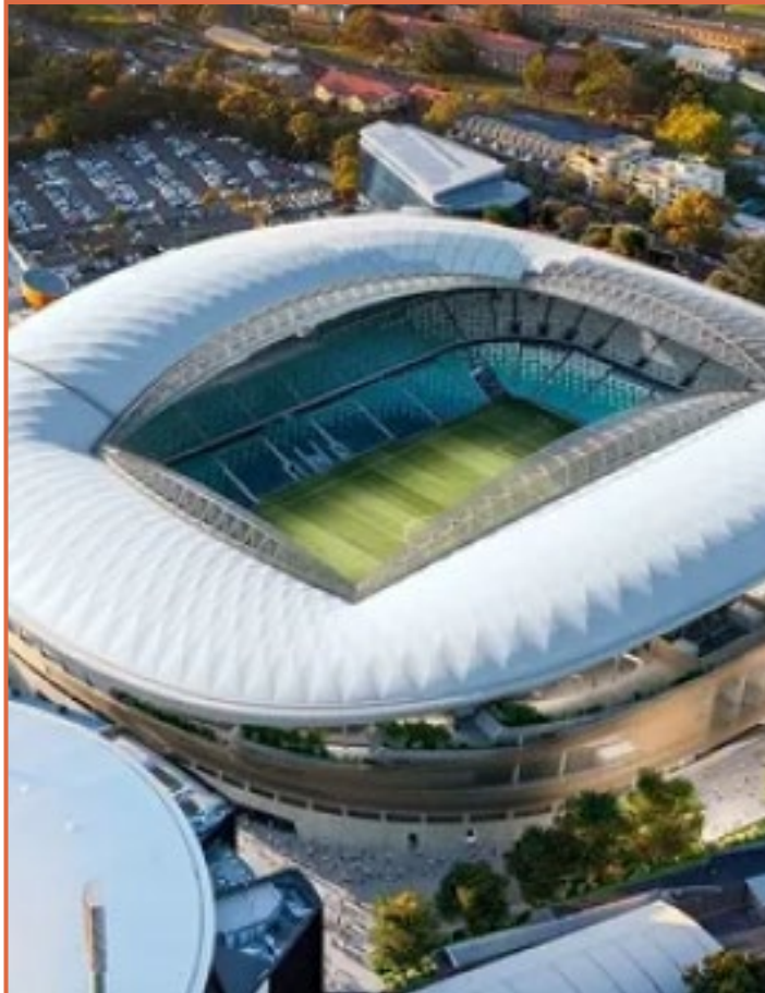
Sydney Football Stadium End of DLP and Defects Closure – Public Asset
