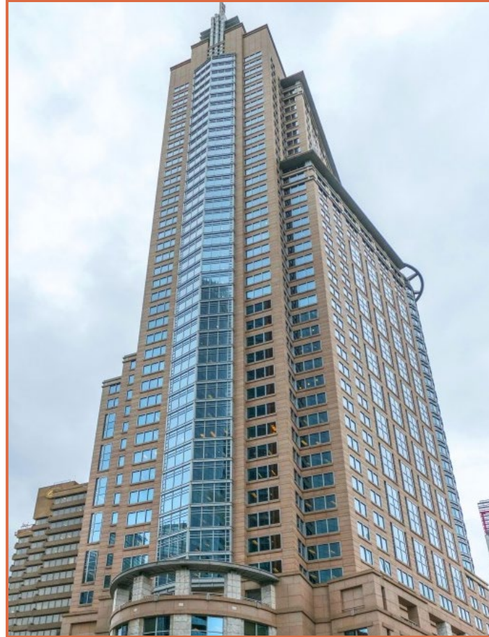
Chifley North Tower | Sydney | Australia Modernisation - Office
