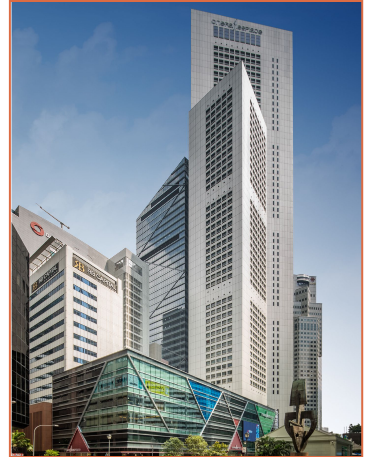
One Raffles Place | Singapore Modernisation
