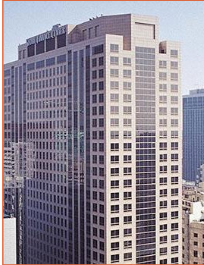
Seoul Financial Centre Modernisation
